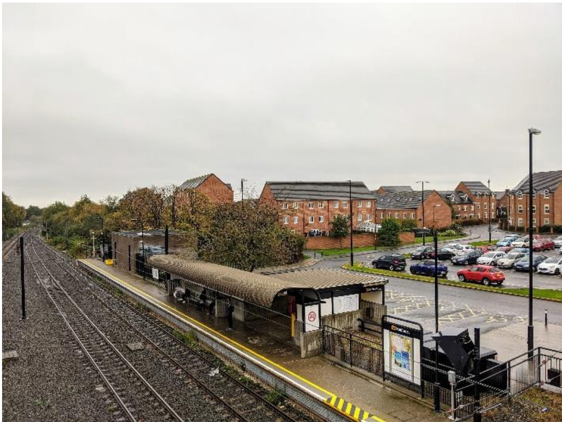
Figure 4.1 Platform 2, which could be rebuilt following the track lowering works
