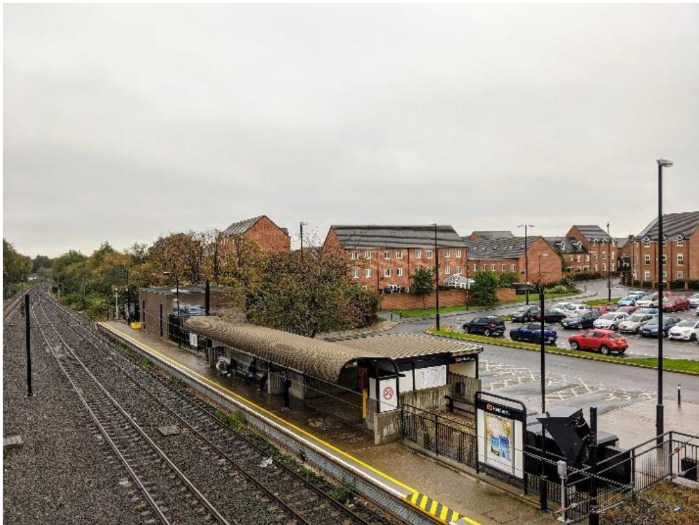
Figure 3.3 Platform 2, Hebburn Metro Station
