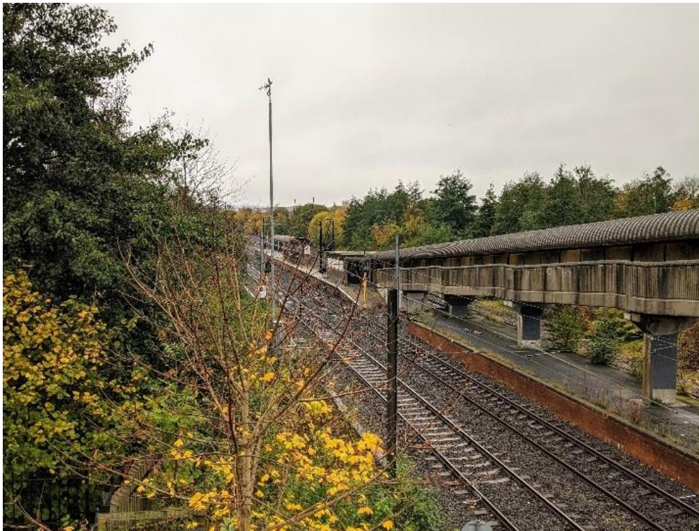
Figure 3.2 Platform 1, Hebburn Metro Station
